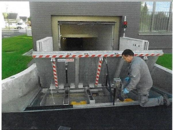
A photograph of a person in a grey uniform kneeling on the ground next to a metal barrier. The person is operating a lever mechanism that is used to lower the barrier. The barrier is currently in an elevated position. The background shows a concrete structure and a green lawn. | <p>Kurbel betätigen und Schott nach unten ziehen</p>                                                               |
